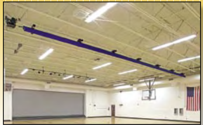
At left: electric winch provided with Fold-Up, Roll-Up, and Top-Roll gym dividers.
